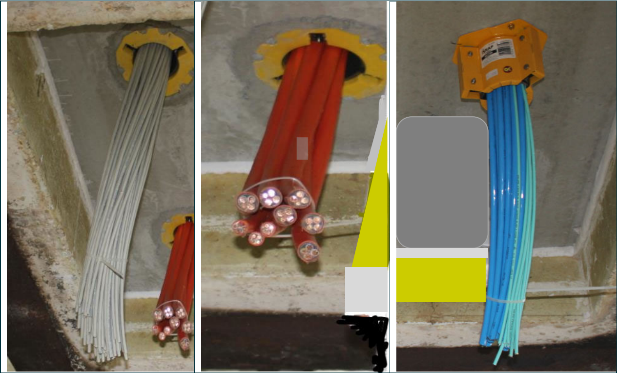
PHOTOGRAPH 1 – EXPOSED FACE OF SPECIMEN 1, 2, AND 5 PRIOR TO TESTING
