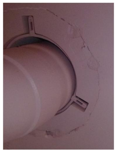
Figure 25c: Thin painted on collar shell and intumescent, refer to Table 17c
